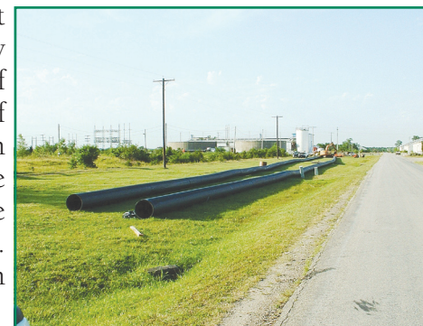
▲ Sections of fused HDPE pipe await installation. Sunflower Water Treatment Plant in background.
