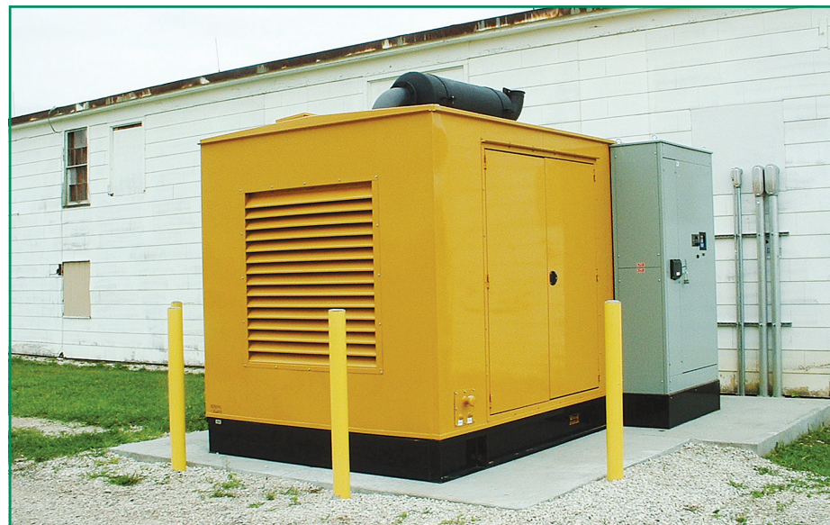
▲ New 350 kW generator at the Sunflower Treatment Plant.
