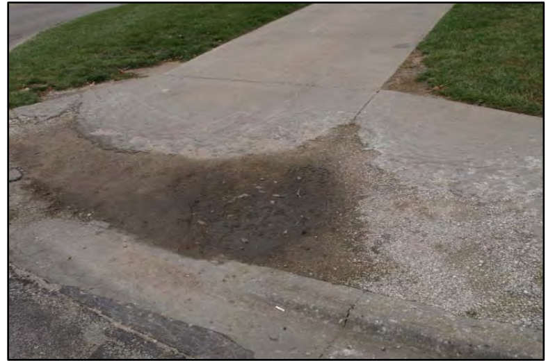
16 – Monticello Trails South Entrance Sidewalk Should be southeast
