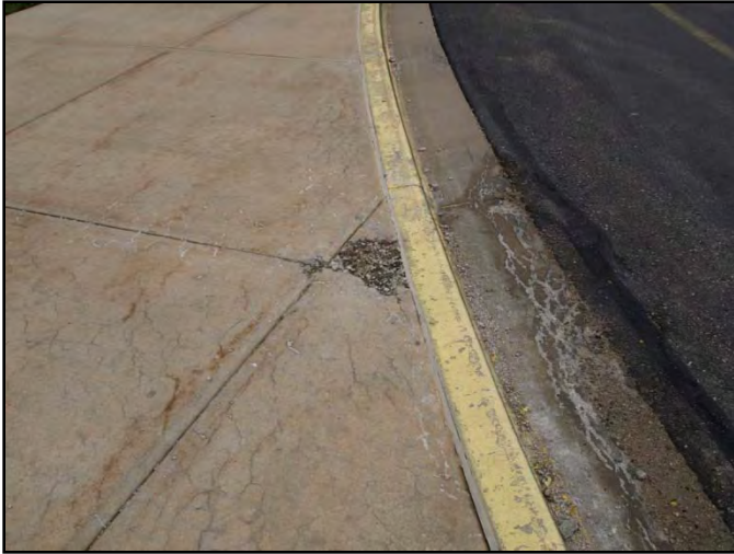
5 – Starside Curb on East Side Front Entrance
