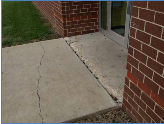
9 – Starside West Wing North Entrance
