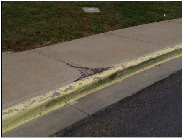
17 – Monticello Trails South Entrance Walk
