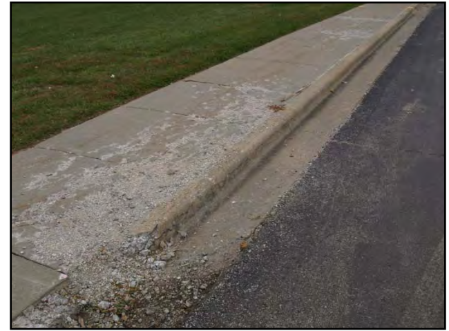
18 – Monticello Trails Sidewalk/Curb South Entrance
