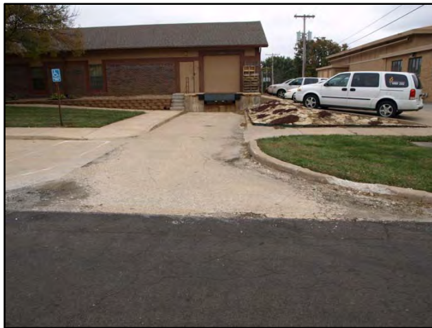
11 – Technology Center Receiving Curb
