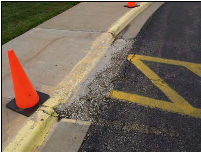
7 – Starside Crosswalk East Side Front Entrance
