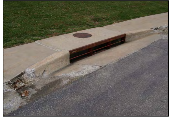
14 – Monticello Trails Should be East West Curb
