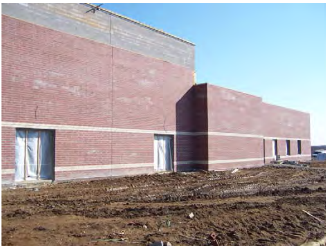
Area A – West Elevation looking South
