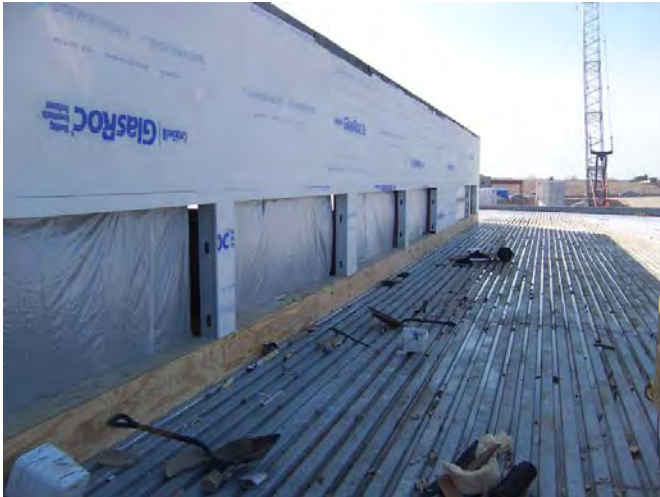
Area C – Activity Area clerestory windows.
