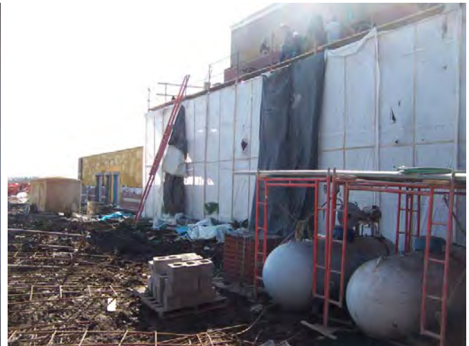
Area A – East Elevation looking South
