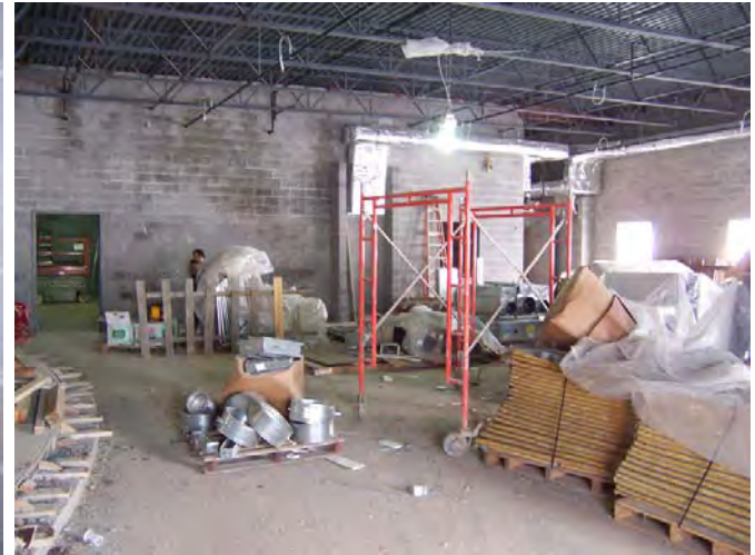
Area A – Cafeteria A117 looking Southeast.
