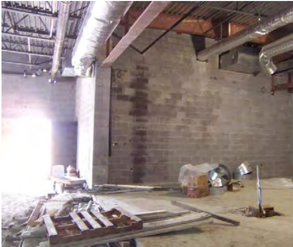
Area A – Cafeteria A117 looking North towards Stage
