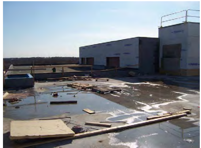
Area B – Roofing installation above Discovery Classrooms
