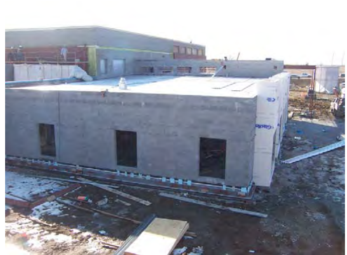
Area D Roofing – Looking down from Area C roof
