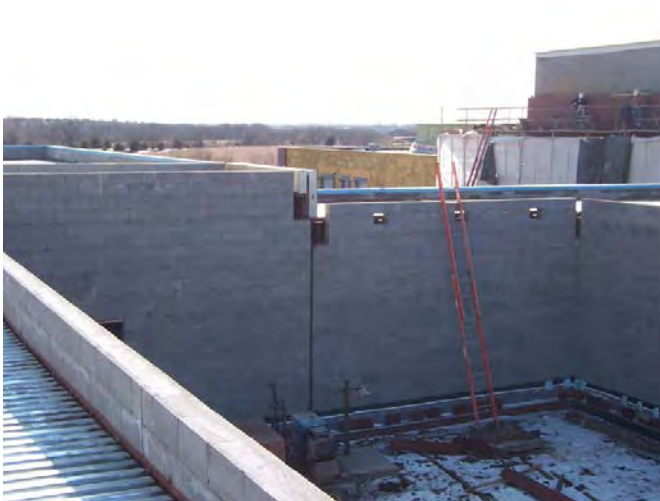
Area D/C roofing transition from Area C roof, looking South
