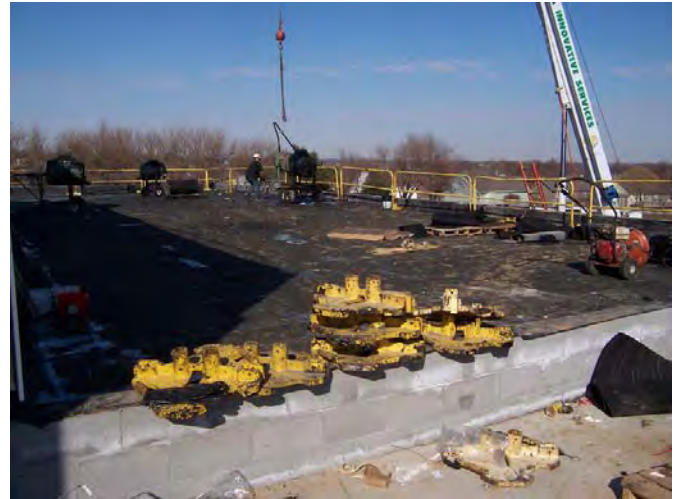
Area C – Roofing installation above Classrooms C239 & C243
