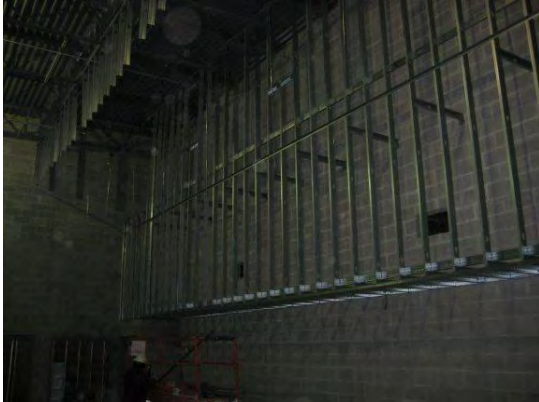
Photo 3: New Band Room – soffit framing along corridor
