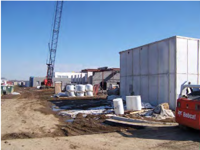
NW Corner of Site looking to the East
