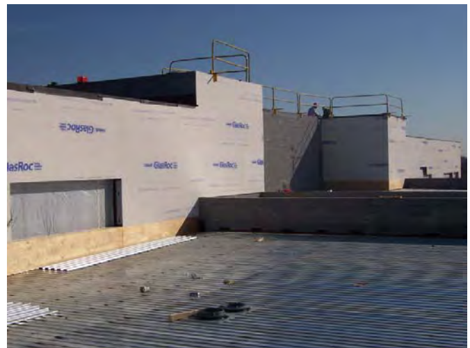
Area B/C roofing transition from Area C roof, looking South
