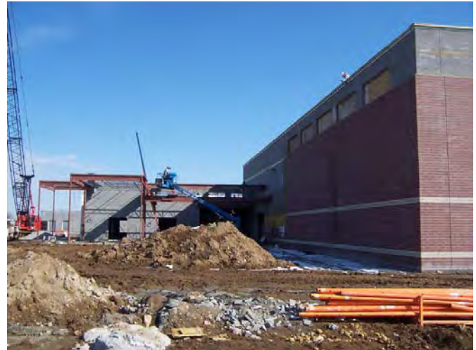
Area A looking East to Area D – Main Entrance to building
