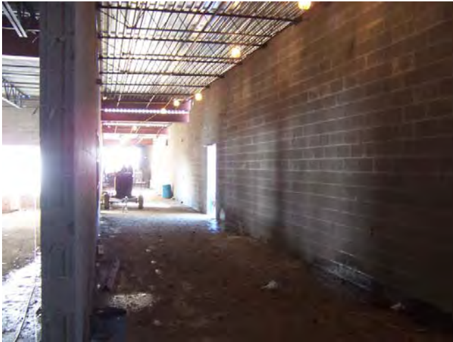
Area B/C – Corridor C207 looking West toward Area D
