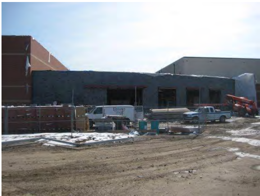
Photo 2: New Event Lobby with completed accent brick
