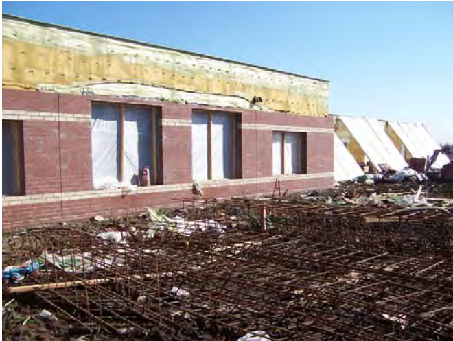
Area B – Media Center, West elevation looking South
