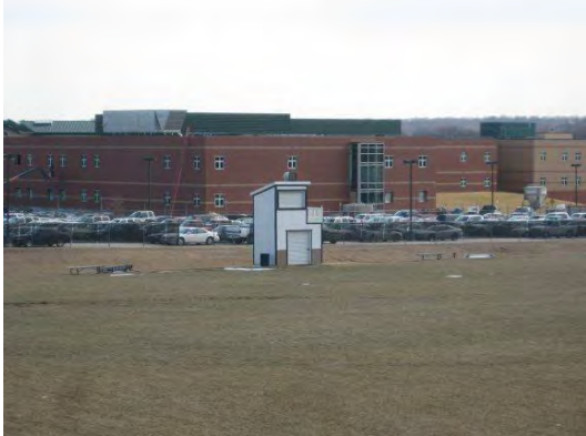
Photo 1: "B" wing exterior fully bricked and windows set
