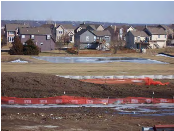
East retention basin from Area B roof looking East
