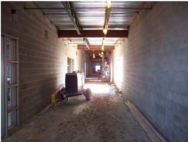
Area D – Corridor D259 looking East towards Areas B/C
