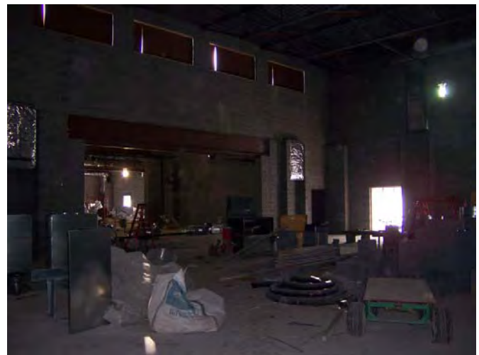
Area A – Gymnasium A101 looking South at Stage
