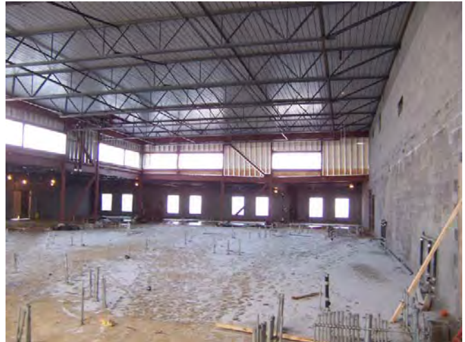
Area C – Activity Areas looking East
