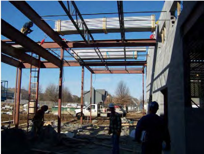
Area D – Corridor D258 looking North – Main Entrance
