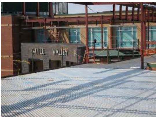
Photo 5: Steel frame at existing Main Entry
