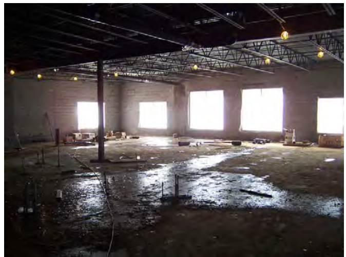
Area B – Media Center B132 looking West
