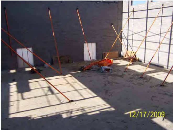
Area A – Gym looking from Mechanical Mezzanine
