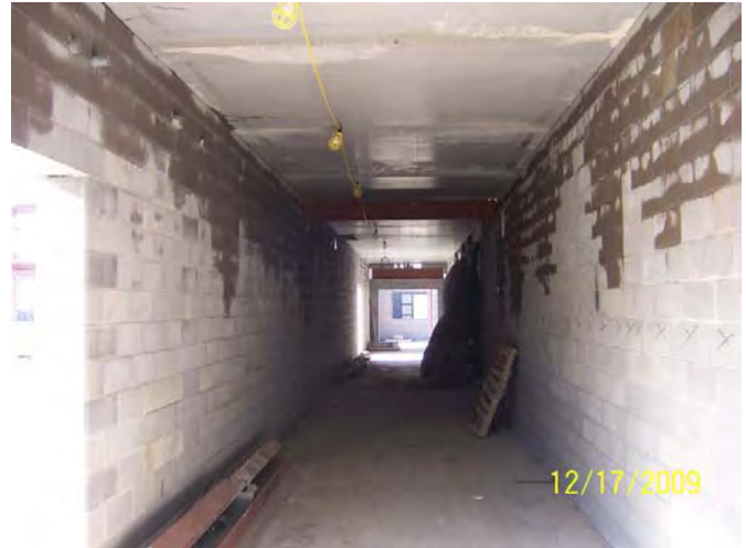
Area B – Corridor B158 looking East
