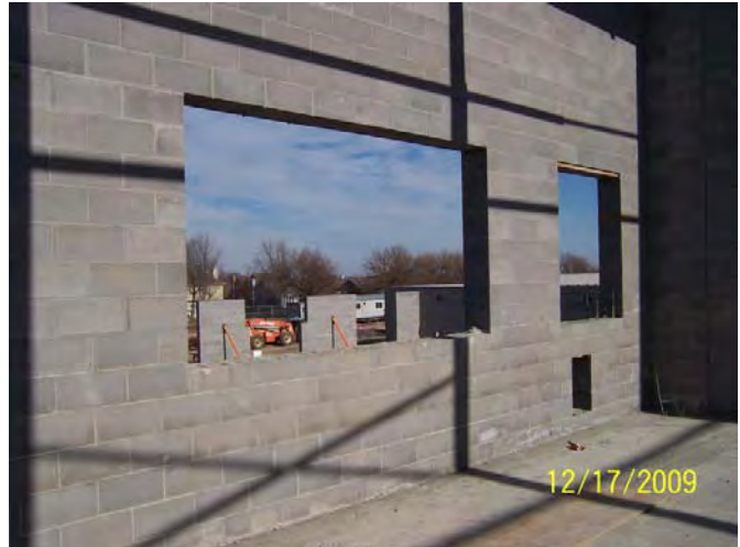
Area A – West opening into Mechanical Mezzanine
