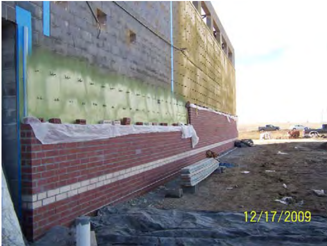
Area A – North Elevation – Brick Veneer installation
