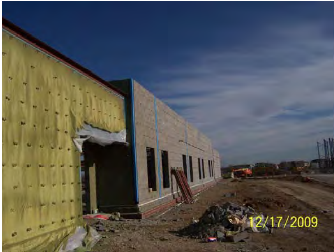
Area B – South Elevation looking East
