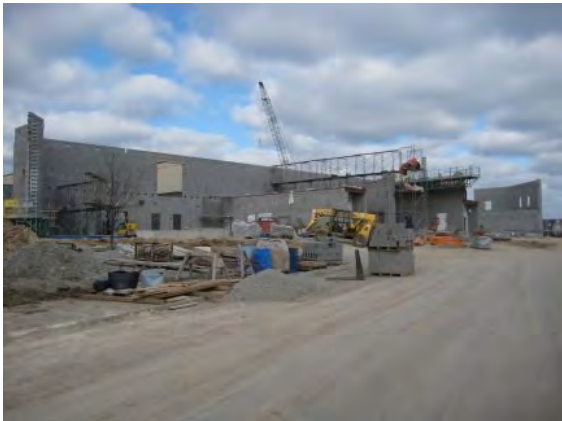
Photo 5: Construction going on around the two permanent Corridors on the front of the building
