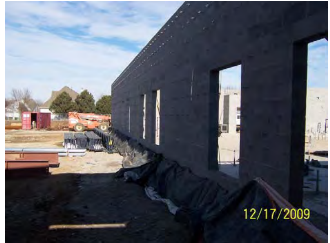
Area C – West Elevation looking North
