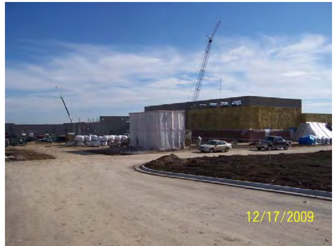
Northwest corner of site looking back at building.
