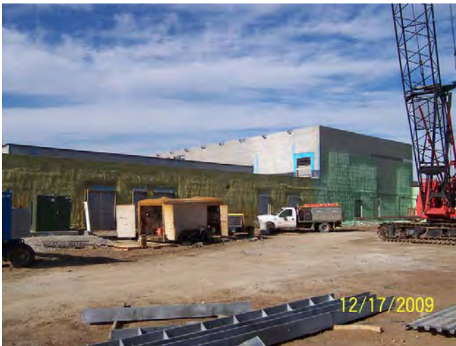
Area A – East Elevation looking Northwest
