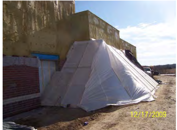
Area A – West Elevation – Cold weather protection for Brick
