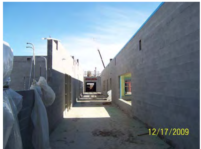
Area D – Corridor D259 looking West
