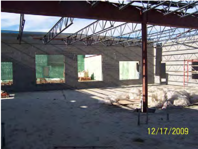
Area B – Media Center B132 looking East
