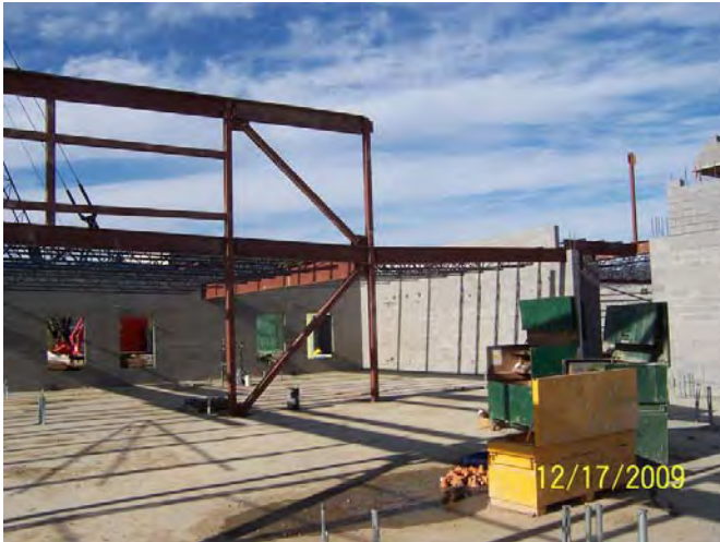
Area B – Structural Steel installation looking Northwest
