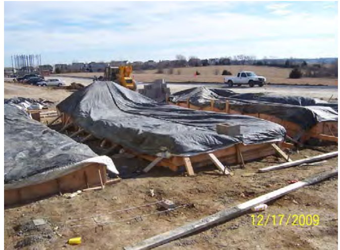
Area A – Exterior mechanical yard – pad installation
