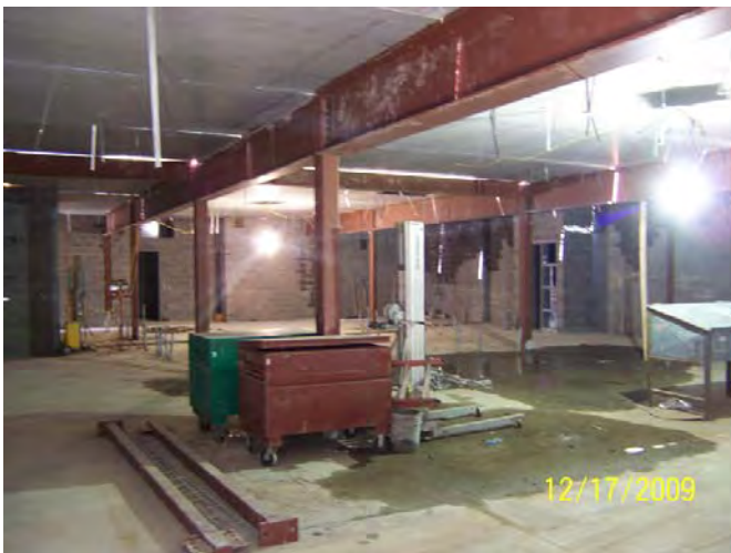
Area B – Discovery Area looking Southeast
