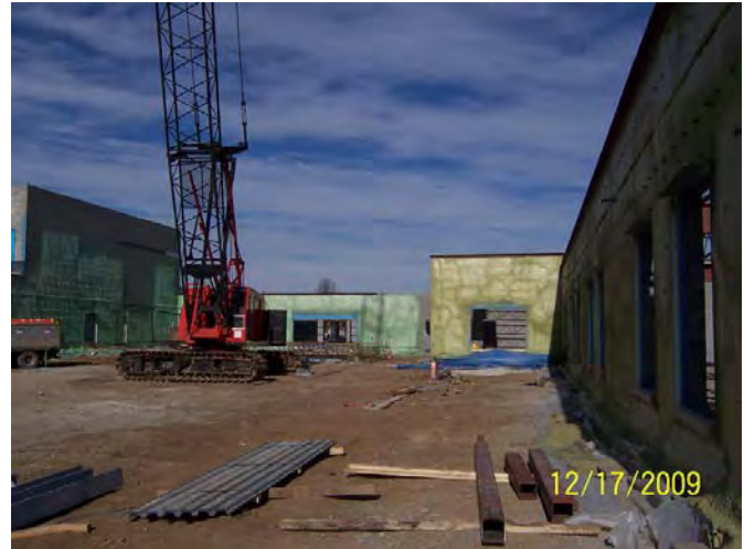
Areas A & B – South Elevations looking North
