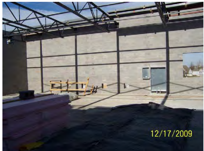
Area A – Mechanical Mezzanine
