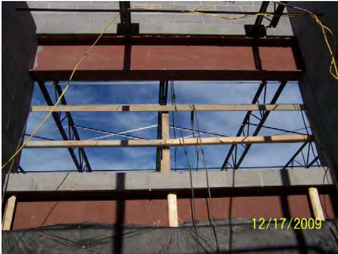
Area A – South opening into Mechanical Mezzanine
