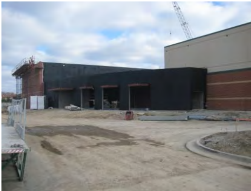
Photo 2: The Event Lobby with applied air barrier
