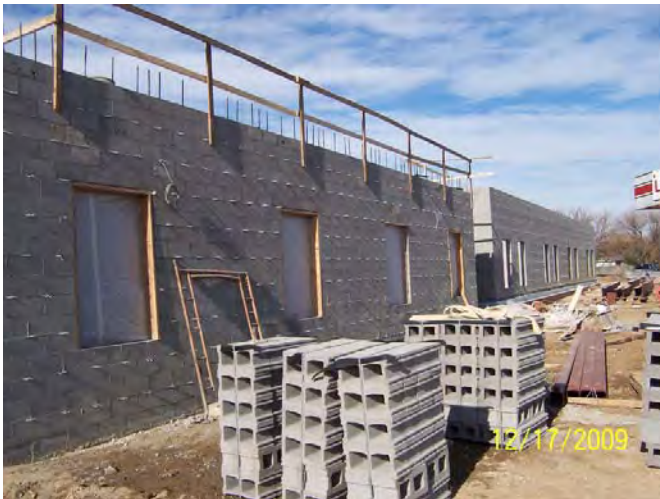
Area B – Alternate Classrooms – East Elevation looking N.
