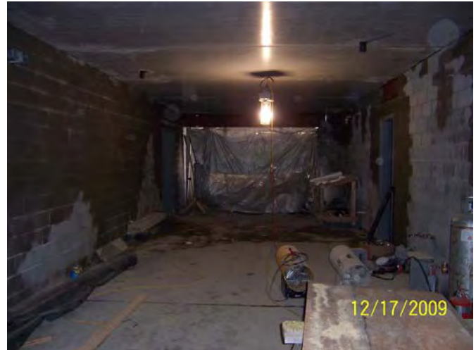
Area A – Corridor A100 – Weather protection installation
