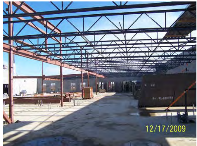
Area B – Structural Steel installation looking East
