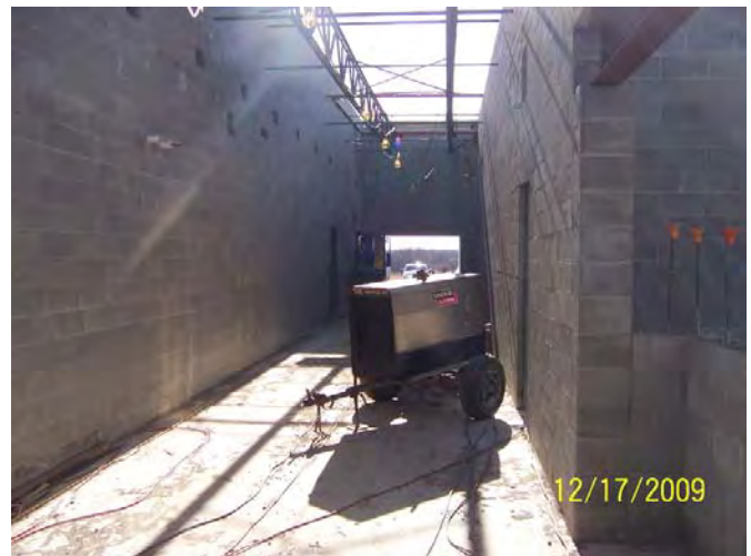
Area A – Corridor A100 looking South
