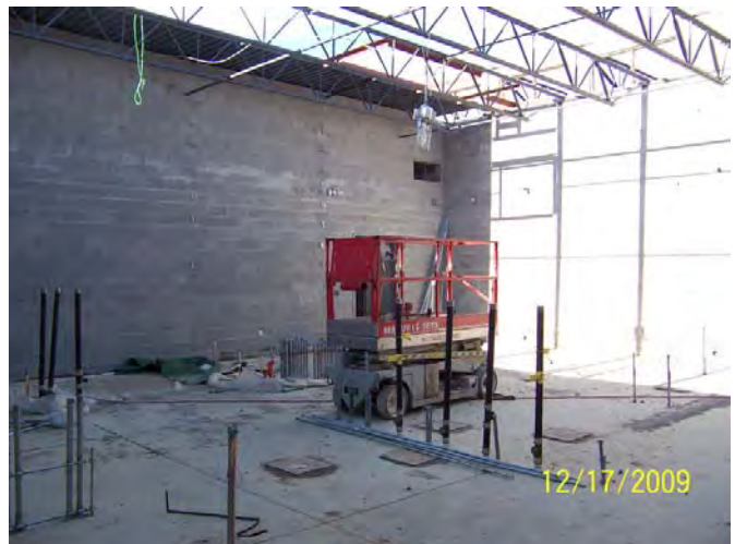
Area A – Kitchen suite looking Northeast
